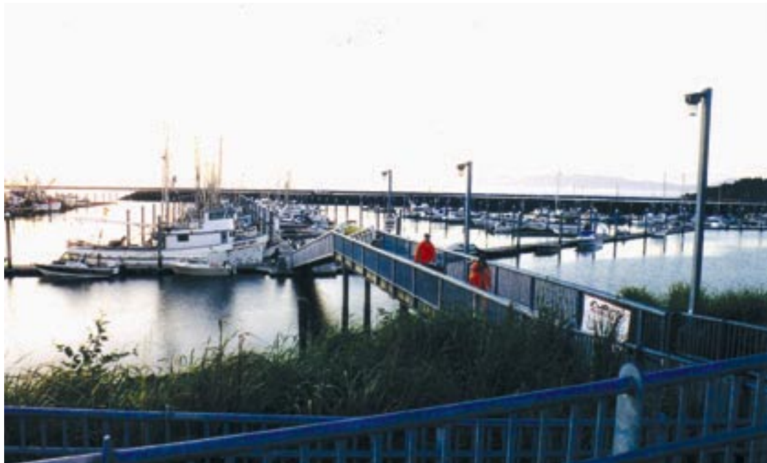
The single largest Initiative investment in Neah Bay was the construction of the Makah Marina.
