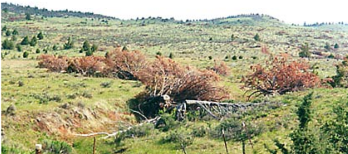
A Jobs-in-the-Woods project that uses cut-down trees to stabilize stream banks on the Warm Springs Reservation, Oregon.
