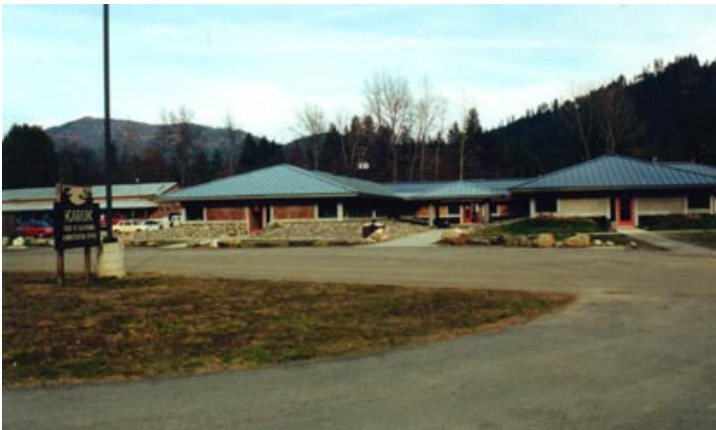
The Karuk Tribal Administration Office houses the governmental facilities of the Karuk tribe.
