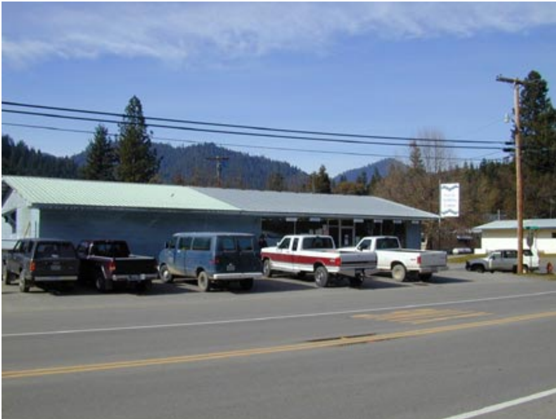
The Karuk Building Center in Happy Camp, CA.
