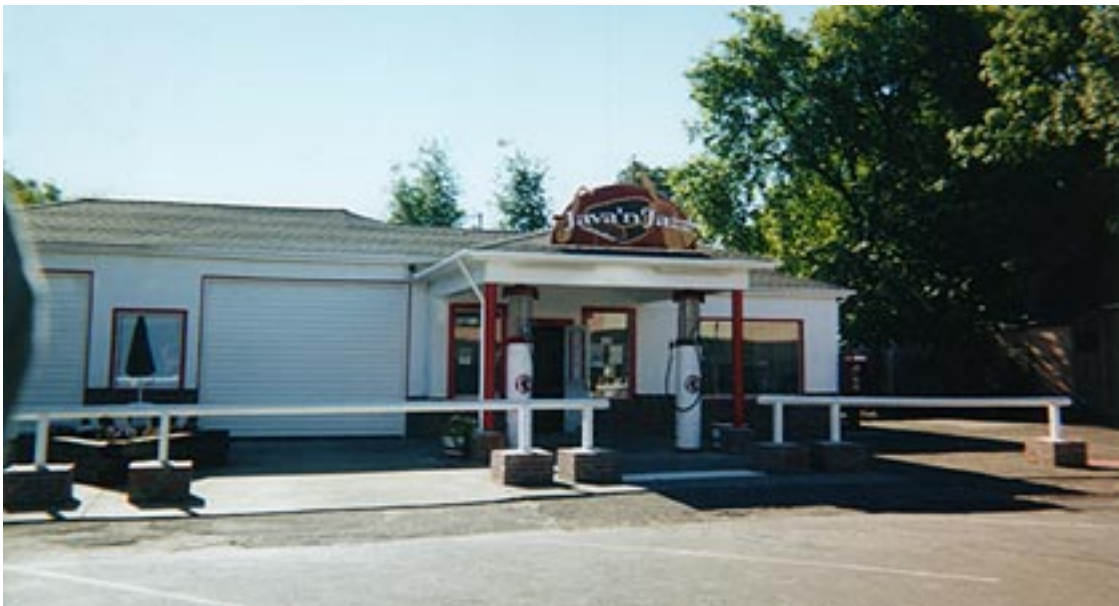
This renovated 1950s gas station has become a coffee shop and a place for music and dialogue.
