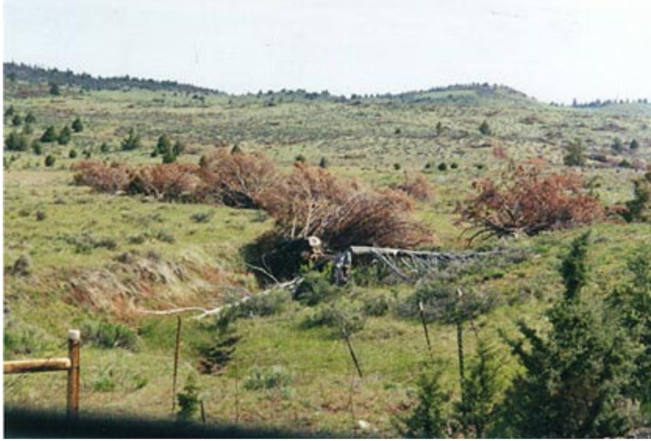
A Jobs-in-the-Woods project that uses cut-down trees to stabilize stream banks.
