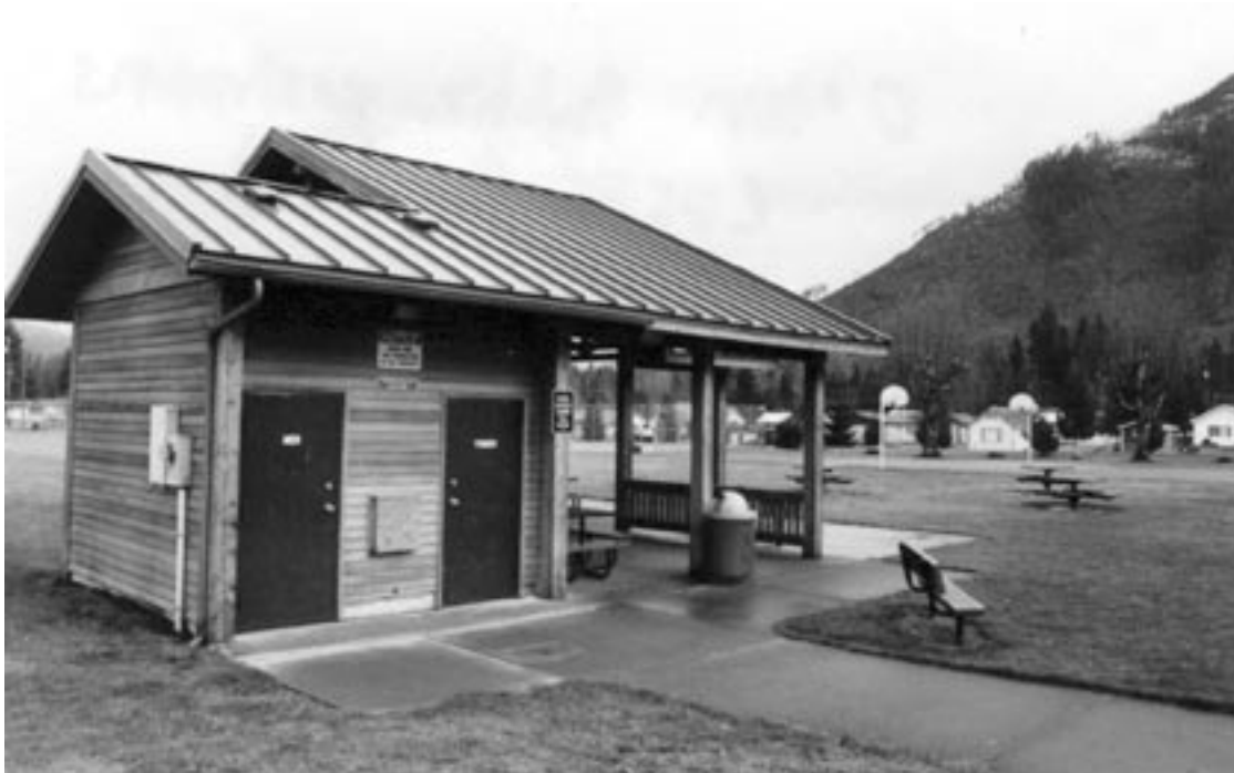
Public restrooms in a park maintained by the city
