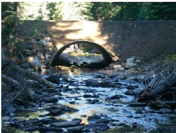
Figure 2. Fish Culvert on Wilson Creek After Replacement
