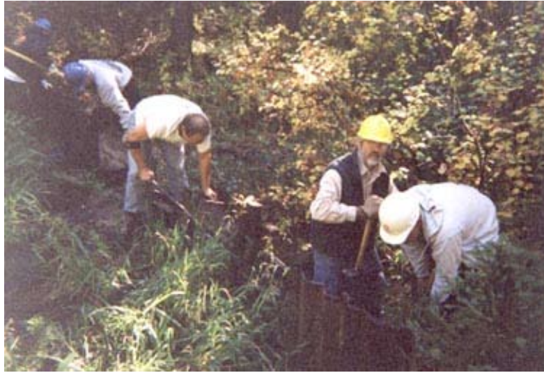
Figure 4. Volunteers Working on the Silver Creek Weir Removal Project
