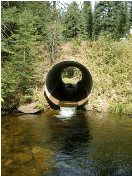
Figure 1. Fish Culvert on Wilson Creek Before Replacement
